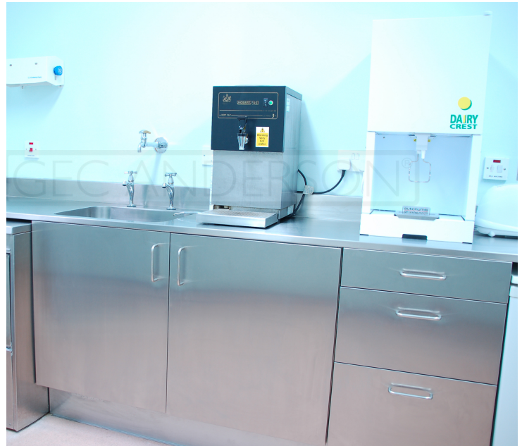
Ward kitchen - sinktop, cabinets and drawers. Wall hung WB45 basin.
