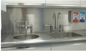
Hand wash and instrument wash sink bowls denoted by shape and fully integrated
