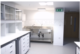
Sinks to restoration rooms
