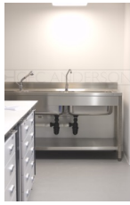
Sinks to restoration rooms
