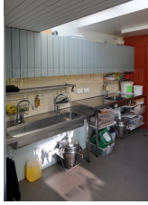
Learning facility sinktop with lowered section and special sink bowls
