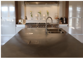
Island worktop with integral sinks, socket outlets and bin chute
