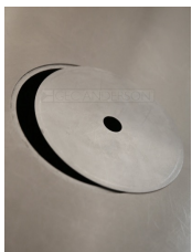
Bin chute and lid with finger-pull hole
