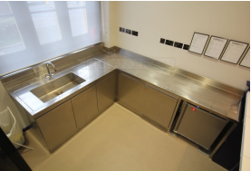
Stainless steel worktop formed in one piece with integral sink and back upstands.
