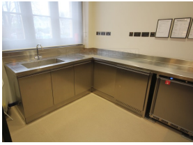
Base cabinets below stainless steel worktop.
