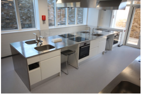
Stainless steel worktops with 20mm edge profile, integral Le50 sinks and cutouts for hobs and electrical outlets
