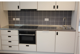
30mm lipped edges (edge 3) with integral sinks and cut out for hob
