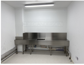
Bespoke sink / worktop with integrated upstand, support legs and front valance
