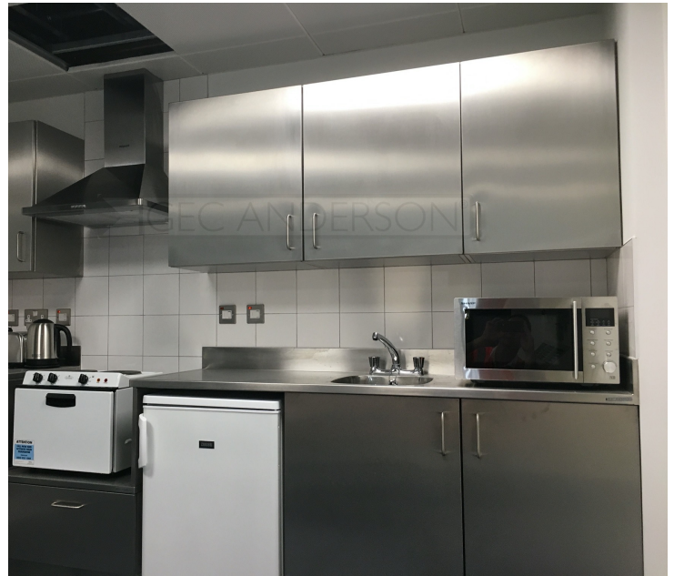
Base cabinets, Baby Belling space, worktops and wall cabinets.
