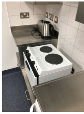
Lipped edge profiles were specified to prevent spillage.
