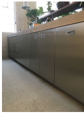
Stainless steel base cabinets with concrete worktop.
