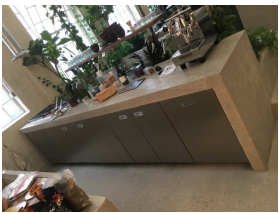
Concrete worktops were cast on site. Stainless steel base cabinets.
